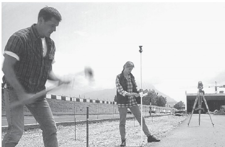
FIGURE 5-36 Leica TPS System 1000, used for roadway stakeout. Surveyor is controlling the remote-controlled total station (TCA 1100) at the prism pole using the RCS 1000 controller together with a radio modem. Assistant is placing steel bar marker at previous set-out point
