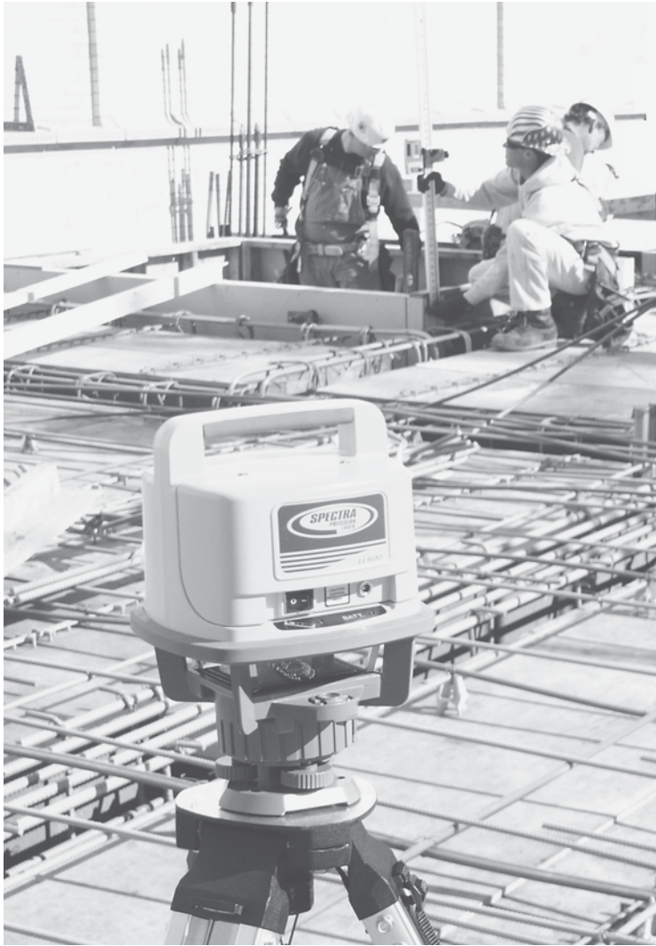
FIGURE 13-41 Spectra precision rotating laser level and an electronic receiver attached to a grade rod, shown being used to set concrete forms to the correct elevation
