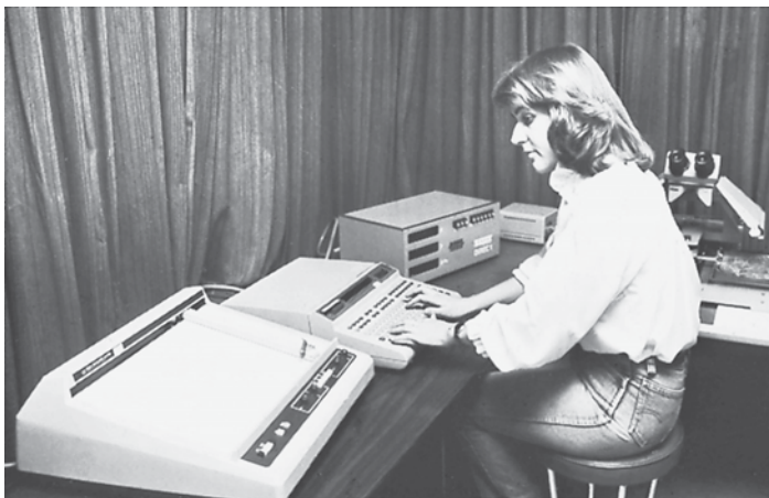
FIGURE 12-10 Computer-assisted plotter for use with photo prints. From left to right: plotter, computer, digitizer, and binocular system for viewing stereoscopic model
